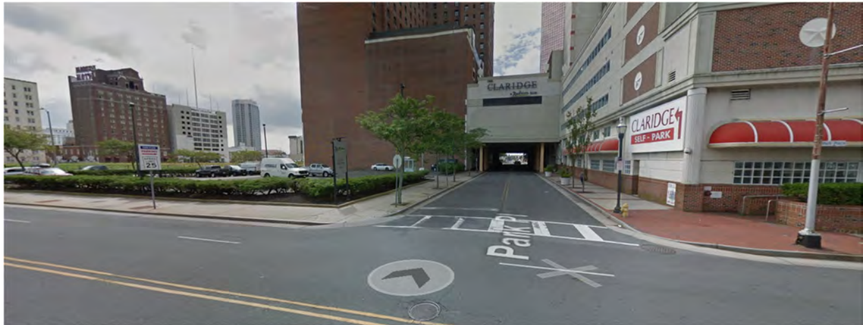
Surface parking lot across Park Place from project site
