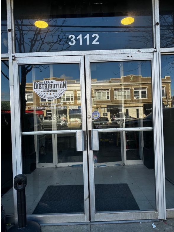
Photo 1 of 3: Vestibule—Double door entry into building on eastern side of Atlantic Avenue
