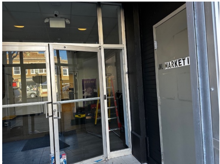
Photo 2 of 3: Vestibule—Second set of double doors walkthrough into ground floor retail dispensary (owner of building)
