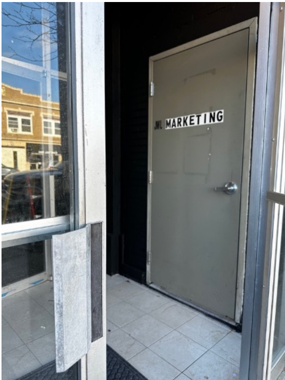
Photo 3 of 3: Vestibule—Southside of vestibule — single and only door to stairwell leading to 2nd and 3rd floors of building.
