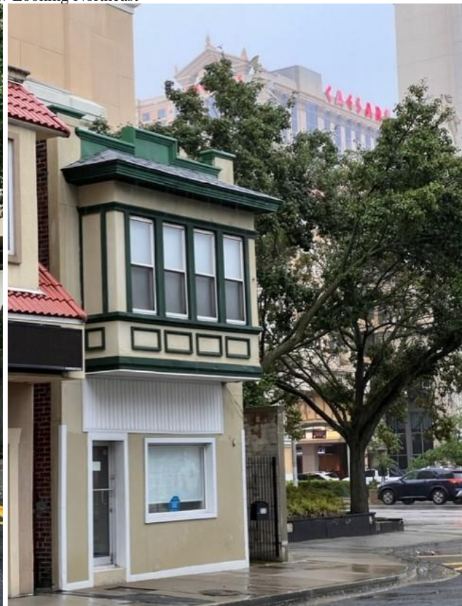
Photo 3 – Site View Looking Southeast
