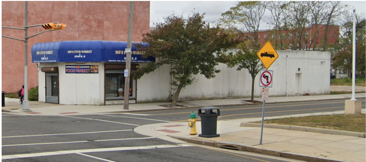
From Atlantic Avenue facing West
