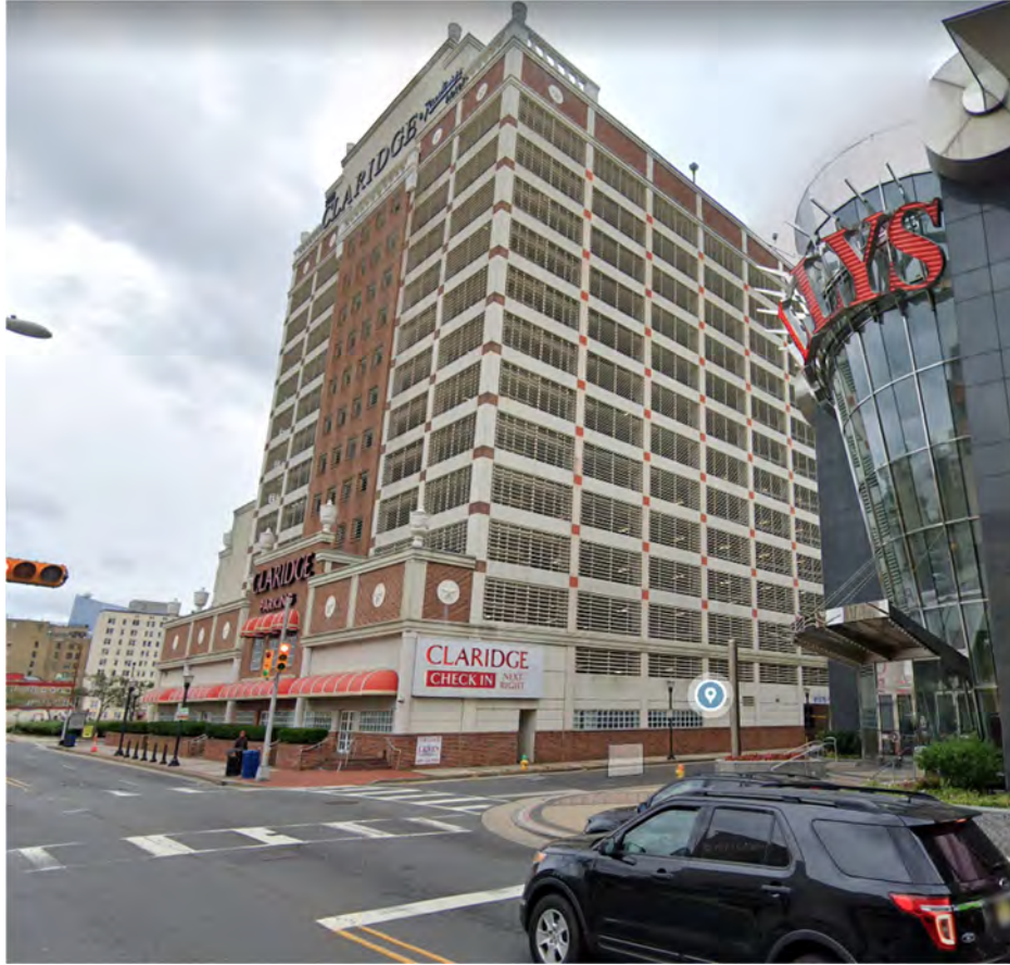
Looking east along Pacific Avenue
