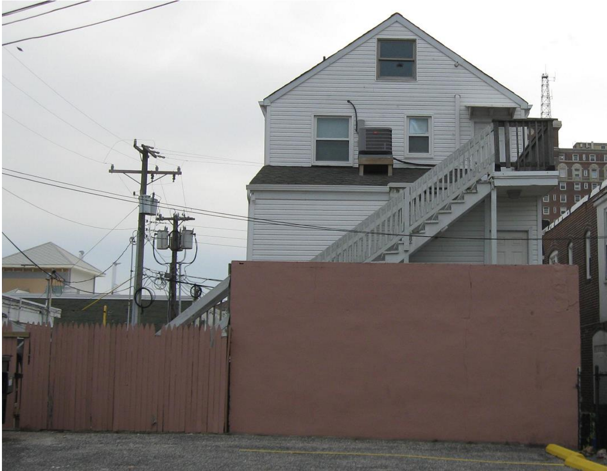
Photo 3 – Site View looking Southeast
