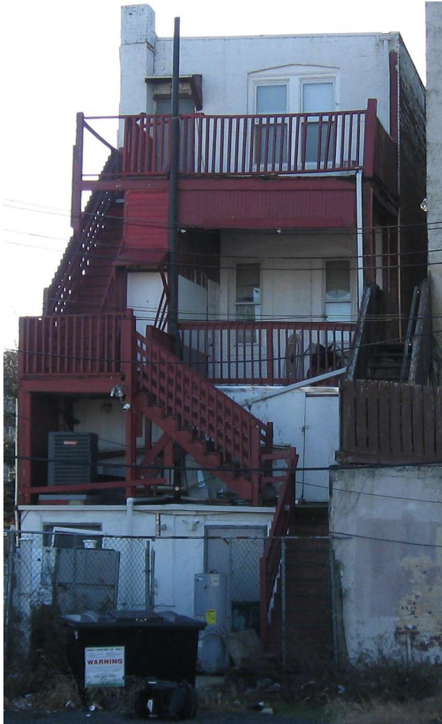
Photo 2 – Site View Looking Southeast
