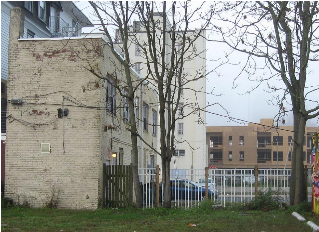
Photo 3 – Site View looking South
