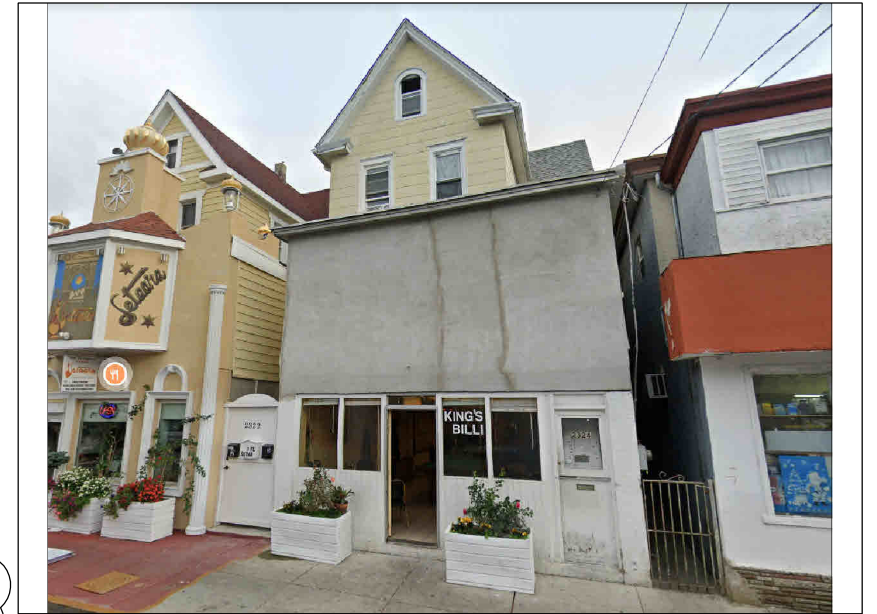
FRONT VIEW (ARCTIC BLDG 2)
